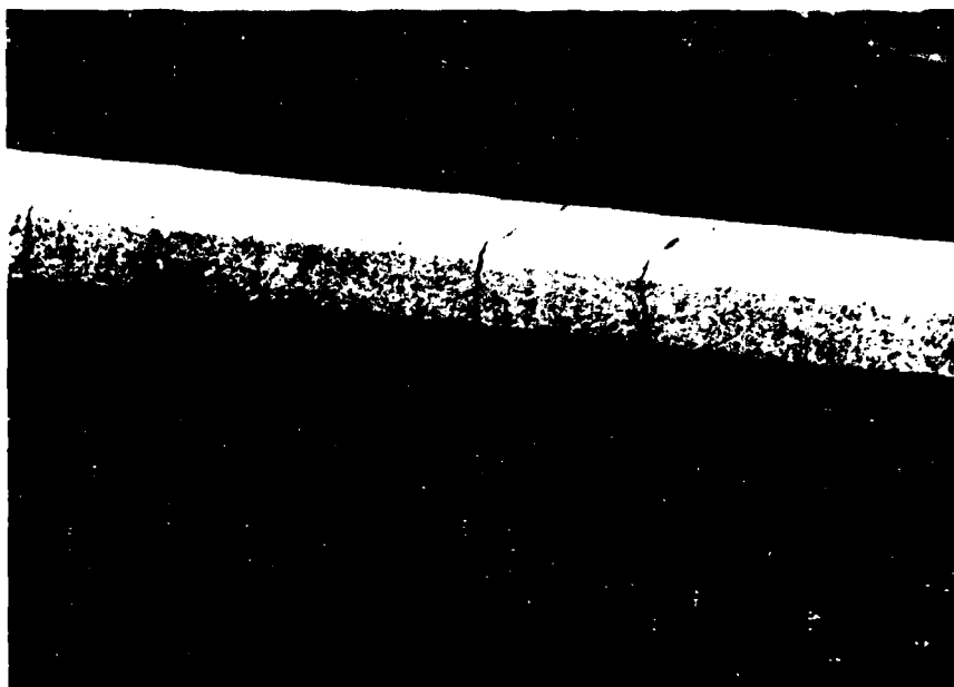
PHOTO #20: Cracks in 12 inch high by 12 inch wide longitudinal sill
