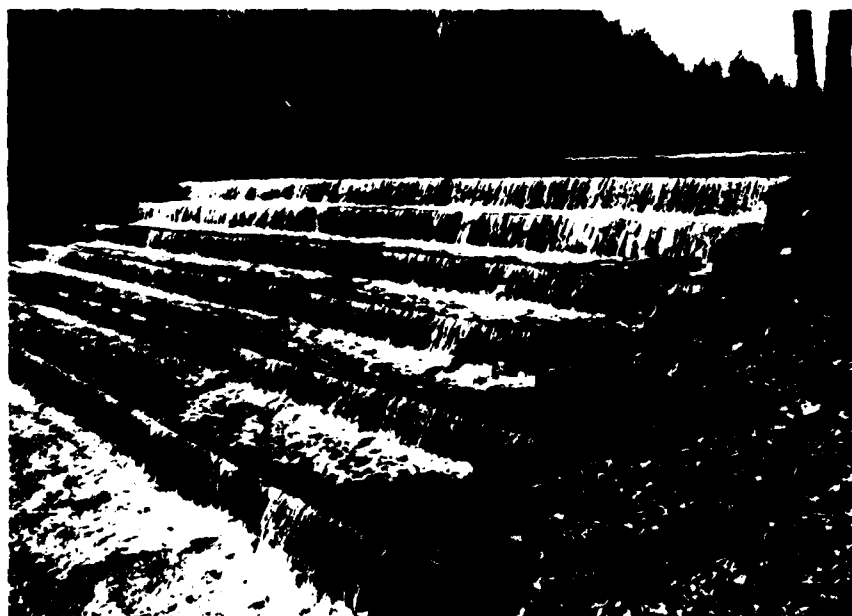
PHOTO #7: Downstream face of dam
