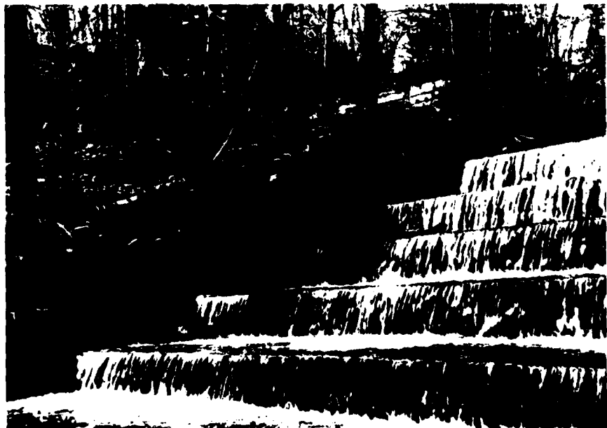
PHOTO #9: Stepped concrete retaining wall on right side of spillway
