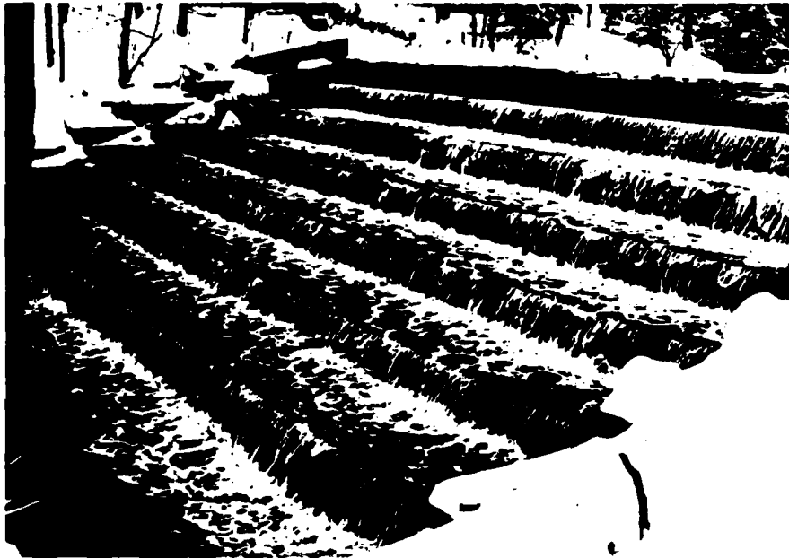
PHOTO #1: Downstream face of dam
