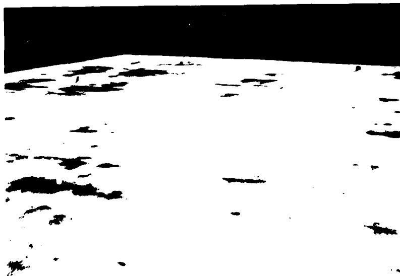
Figure 30. Spots where water had ponded.
