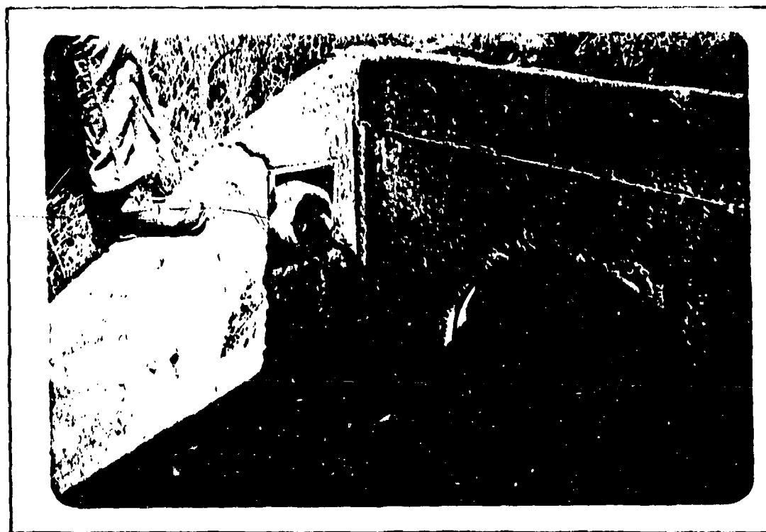
12. CLOSE-UP OF PRINCIPAL SPILLWAY OUTLET STRUCTURE SHOWING CRACKED AND HONEYCOMBED CONCRETE. (4/8/81)
