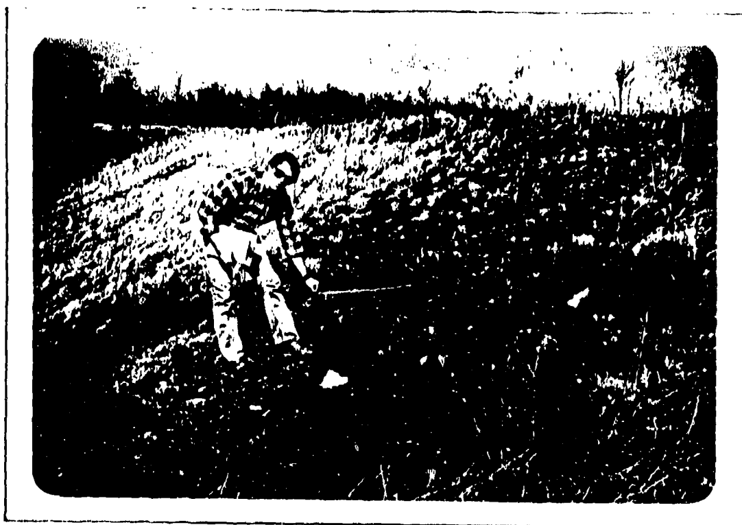
9. SLOPE FAILURE IN THE DOWNSTREAM FACE OF THE DAM. (4/8/81)
