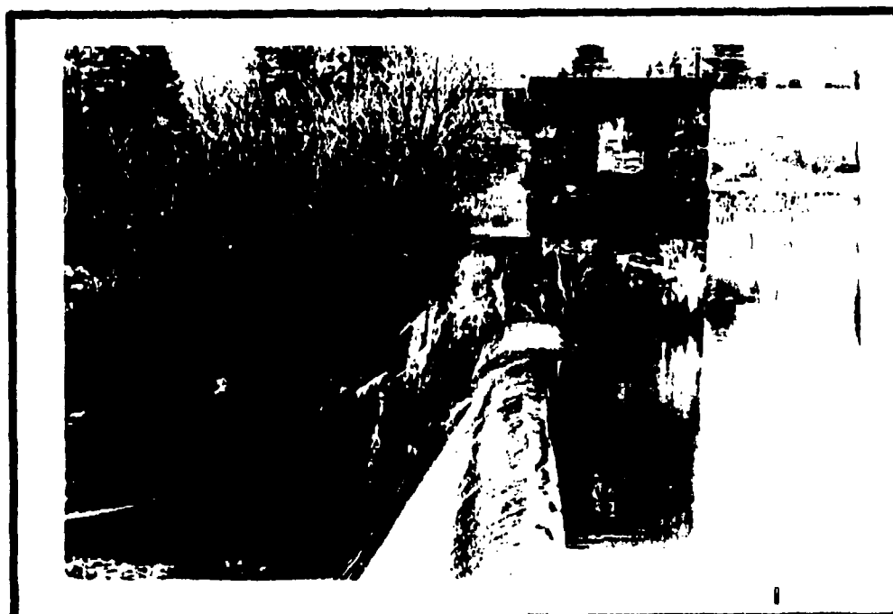
LOW FLOW NOTCH IN SPILLWAY - NO. 7
