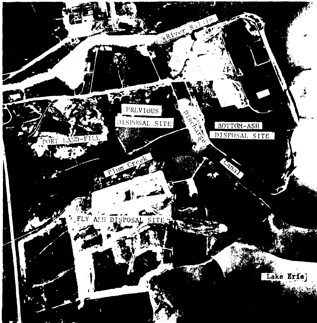
Fig 3 Aerial photograph of the Monroe area, 1975.
