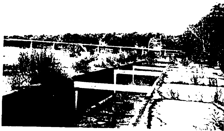
PHOTO 4: SPILLWAY AND CHANNEL (LOOKING UPSTREAM)
