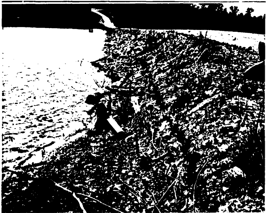
PHOTO 6B: Wavewash on Upstream Embankment
