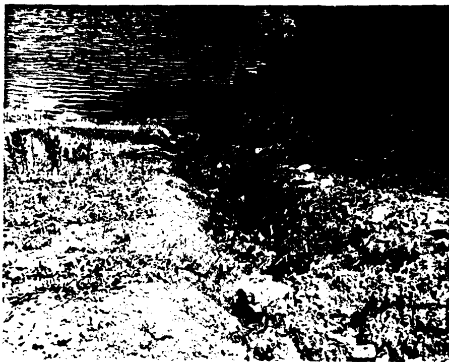
PHOTO 7B: Erosion Gully in Upstream Embankment near Left Abutment
