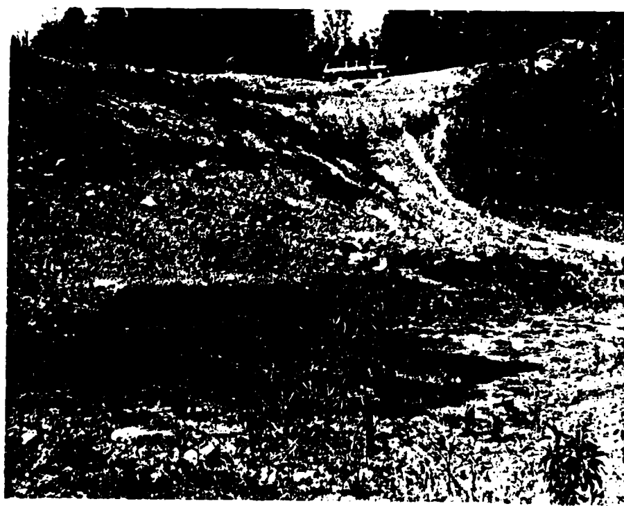
PHOTO 12D: Wet Spot at Toe of Dam
