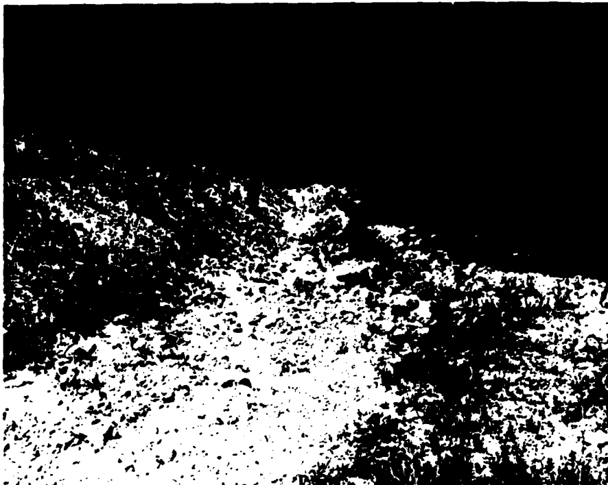
PHOTO 7E: Erosion Gulley in Downstream Embankment at Left Abutment
