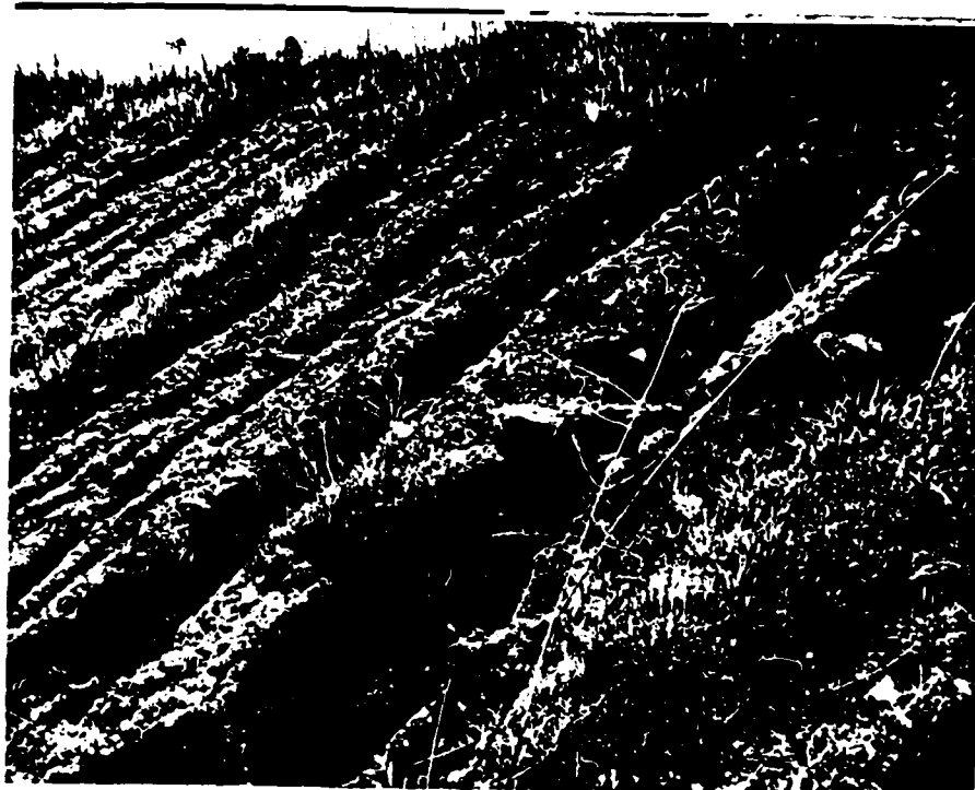
PHOTO 9D: Erosion on Downstream Embankment near Dam Crest
