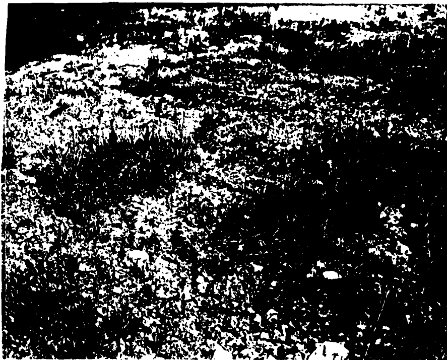
PHOTO 11C: Erosion on Downstream Embankment near Right Abutment
