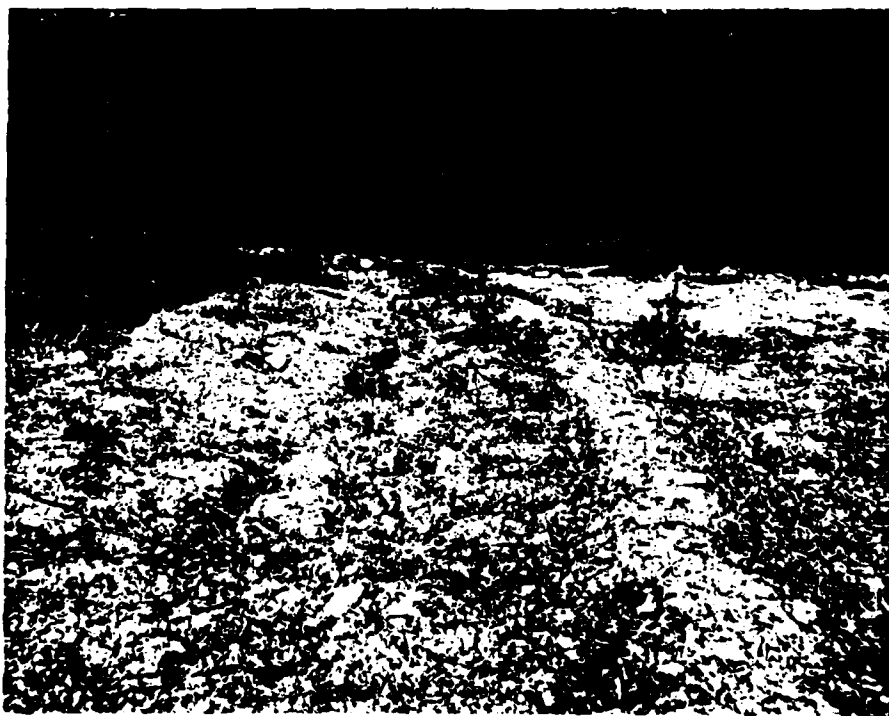
PHOTO 8B: Erosion Gully in Downstream Embankment near Left Abutment
