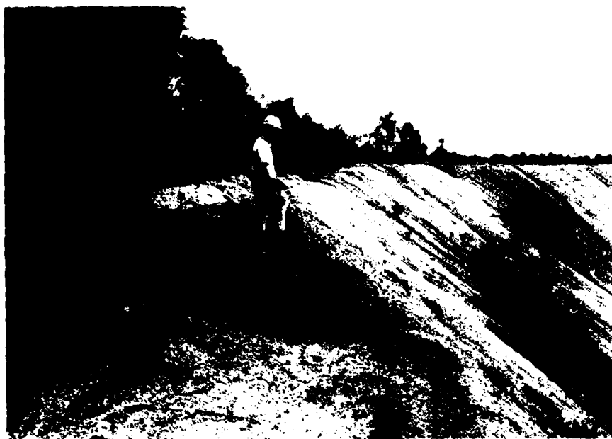
1. End dumped tailings used to construct dam. Looking north along crest.
