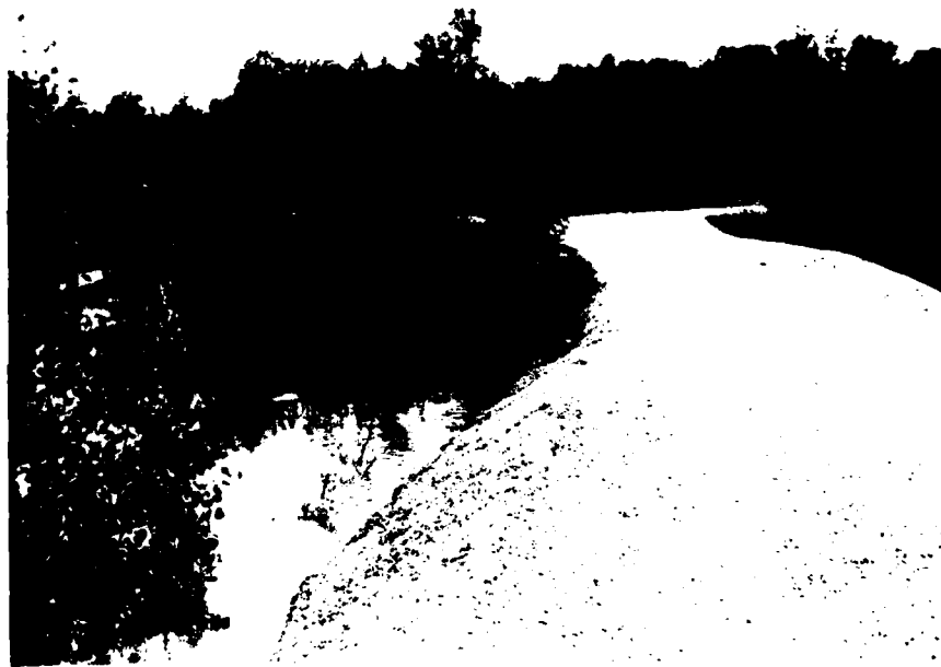
8. Dike along north side of impoundment, showing 1\frac{1}{2} to 2 feet freeboard.
