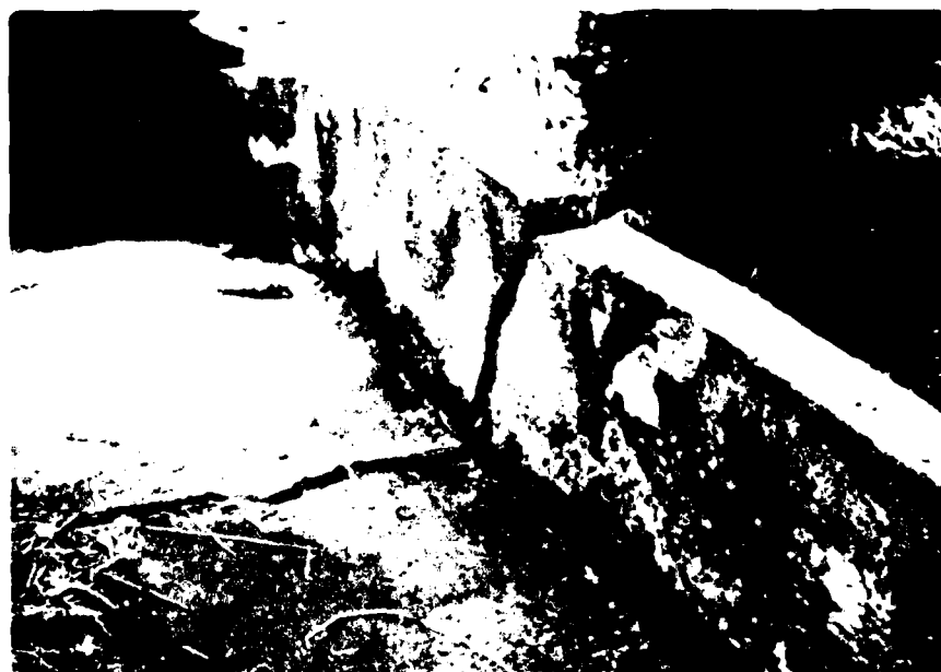
PHOTO 8: DISPLACEMENT OF BOX SPILLWAY CHUTE
