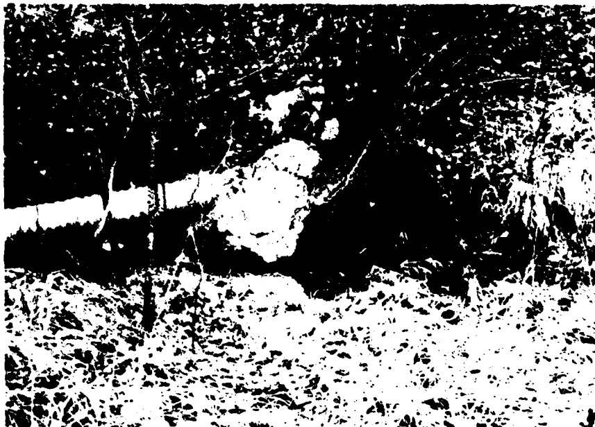
PHOTO 11: DROP INLET SPILLWAY CONDUIT AT DOWNSTREAM TOE
