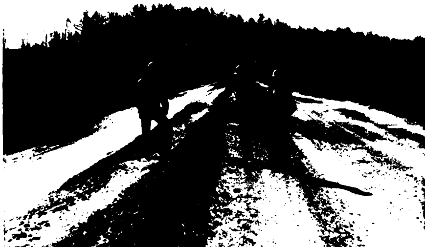
3. Gravel road on crest of dam. Note gravel berms along the shoulders of the road to prevent erosion on the slopes of the dam. Looking southwest from near the center of the dam crest.
