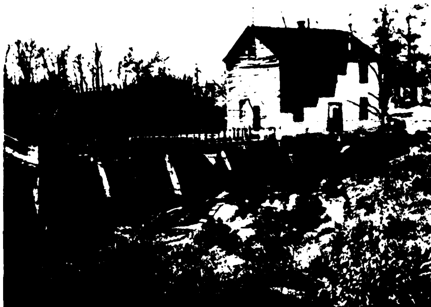
Photograph No. 1 - Overflow Section at Left End of Dam, Catwalk, Turbine House and Mill (Arrow)
