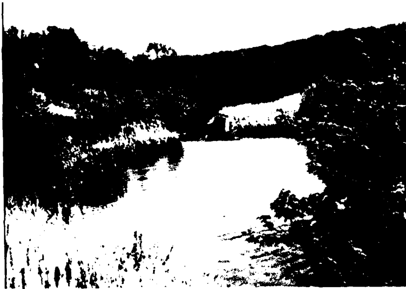
Photograph No. 3 - Approach Channel and Weir
