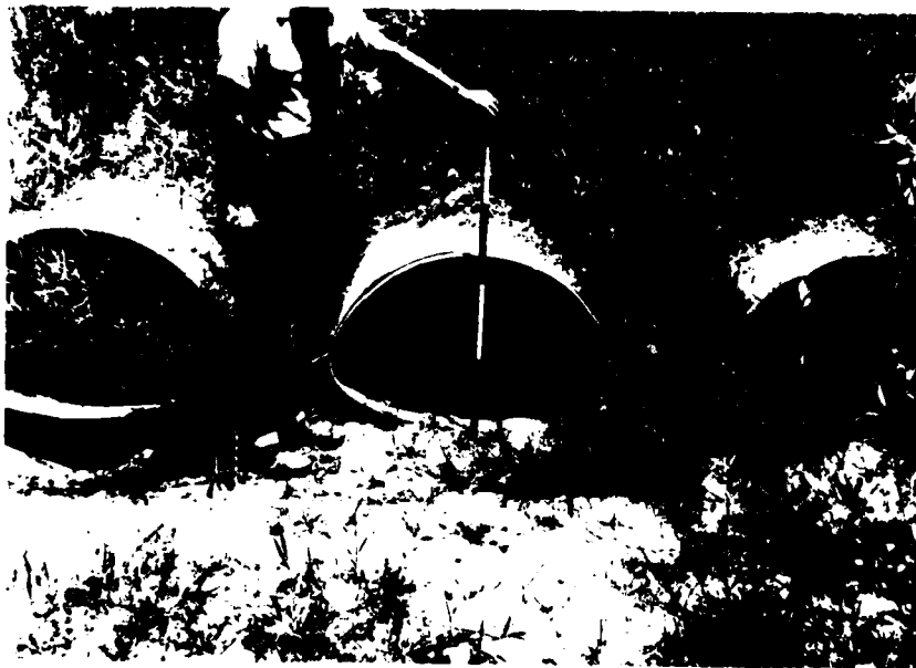
PHOTO 8: OUTLET END OF SPILLWAY PIPES
