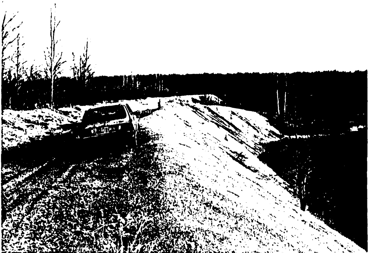
OVERVIEW OF THE EAST END OF THE TAILINGS IMPOUNDMENT OF DRESSER NO. 1 DAM AND DOWNSTREAM POND
