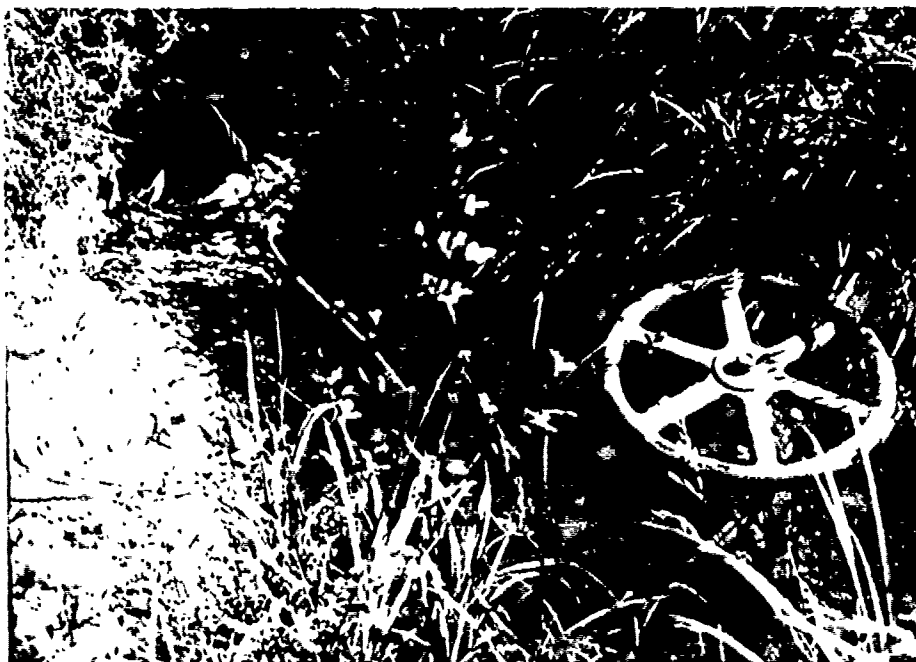
NO. 9: 10" VALVE ON PUMP DISCHARGE LINE
