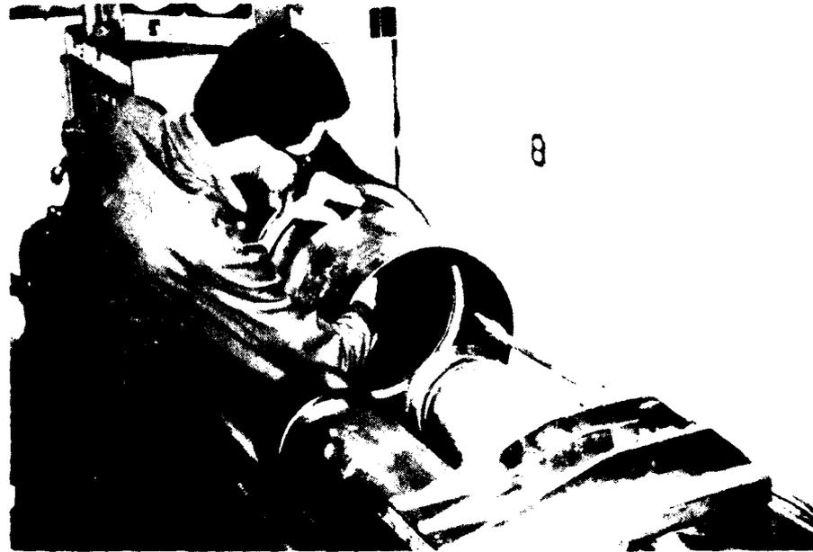
*Figure 53. Thermomechanically treated, internally ribbed tube being removed from the die.*
