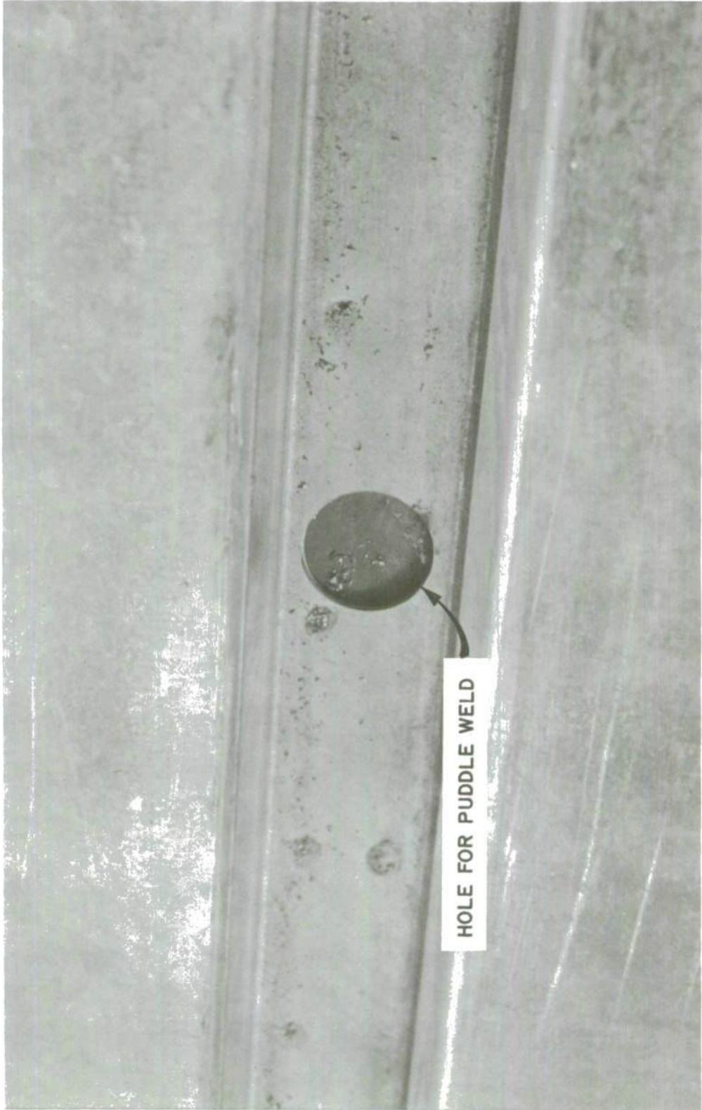
Figure 7. Hole for puddle weld
