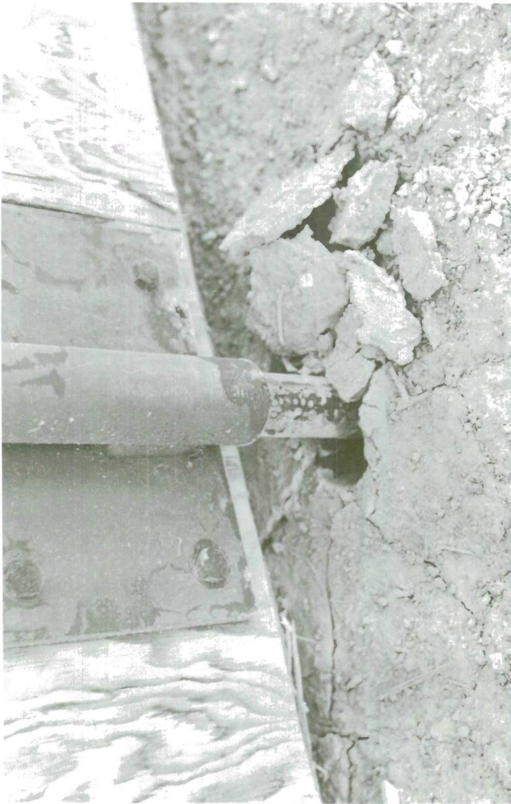
Figure 26. Cracked foundation at Structure B
