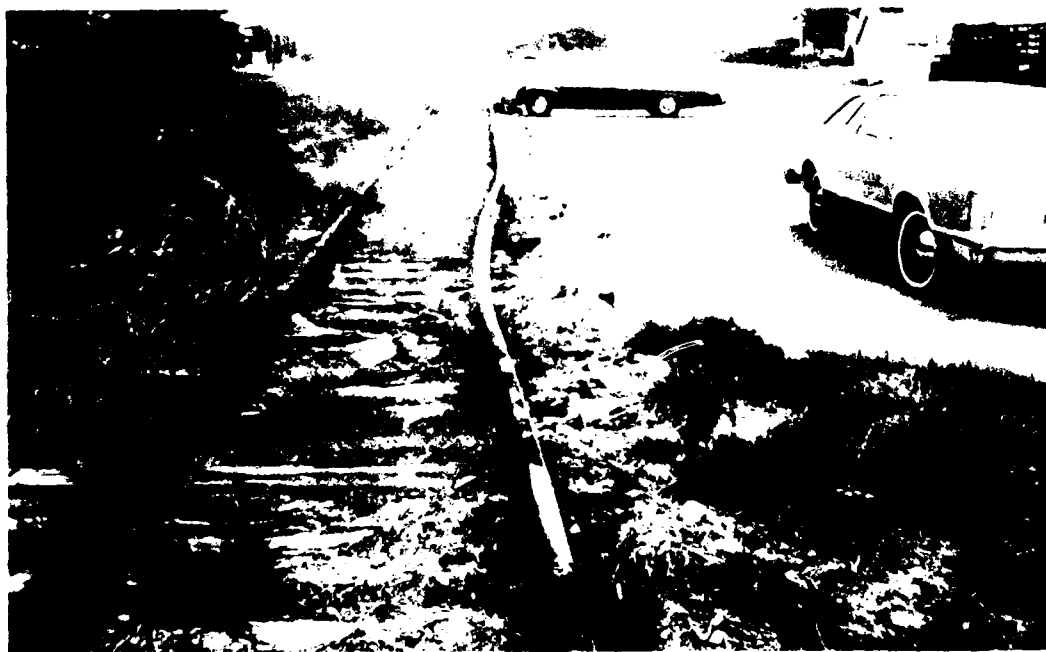
Figure 6. Tank track, snowplow damage.
