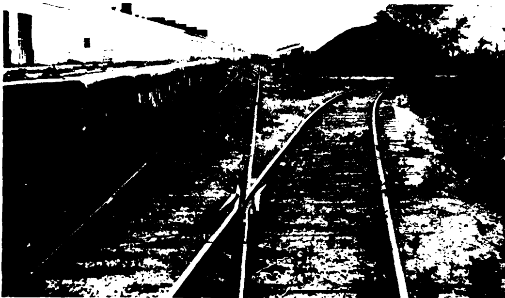
Figure 7. Concrete side ramp, track 1 (left).
