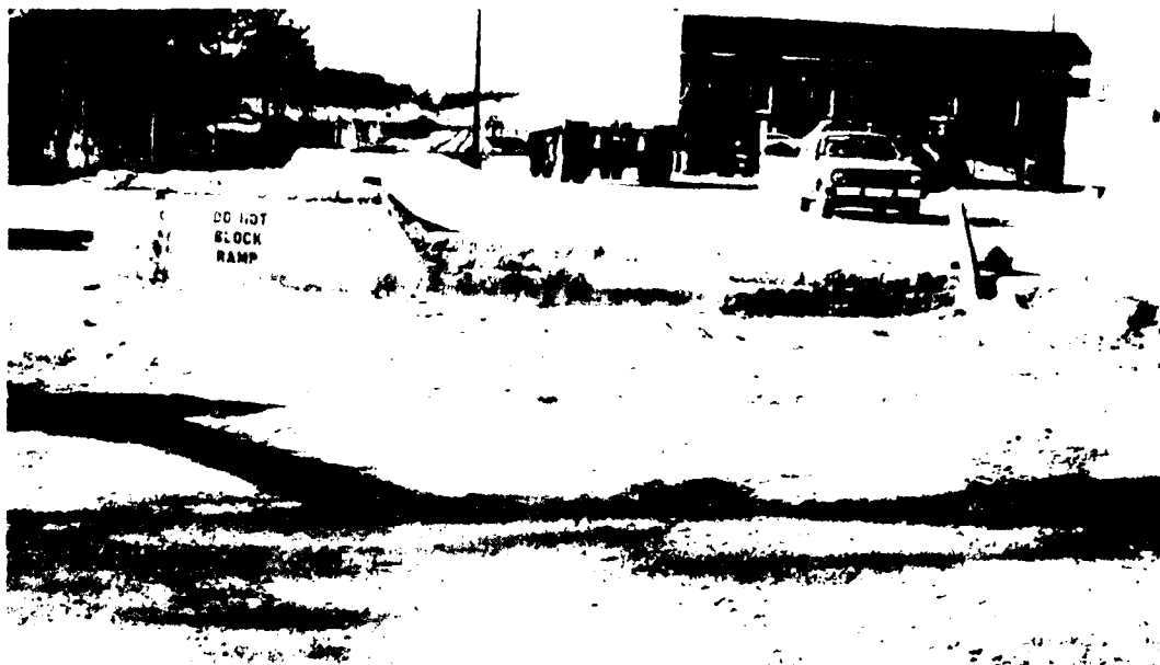
Figure 48. Two-position concrete end-loading ramp.
