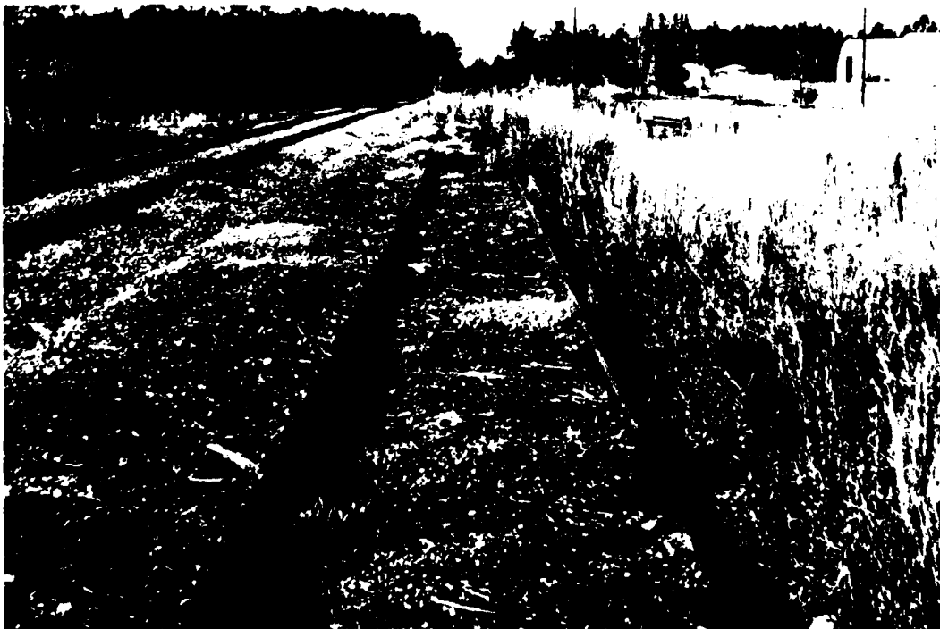
Figure 6. ICG spur L2. (This spur needs maintenance badly. The crossties will soon rot if drainage and weeds are not controlled.)
