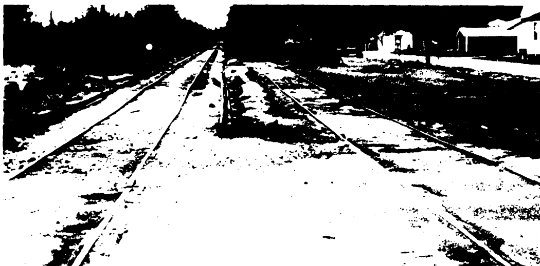
Figure 46. New Augusta siding (looking west). (The siding is to the right and main line to the left. Staging area, to the right of siding is small with a naturally grown surface condition. There is no end ramp nor lighting, and there is 60-pound rail siding.)
