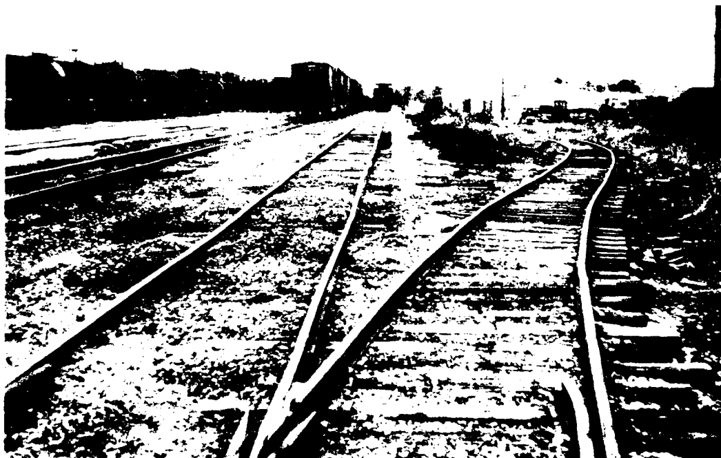
Figure 33. ICG Hattiesburg yard track 4 (looking north). (Track 4, right side of figure, can be used for side and end loading with portable ramps. It has good accessibility from James Street. Vacant lots between track 4 and James Street can serve as staging areas.)
