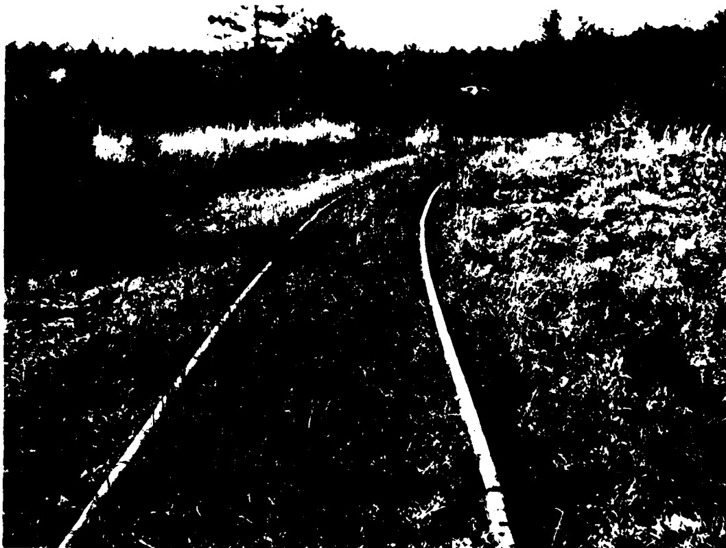
Figure 18. L5, east spur at north end near switch at ICG main line. (Note poor drainage.)
