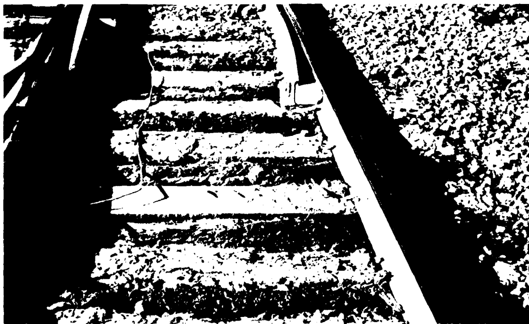
Figure 13. ICG main line at switch to L4. (Mud pumping up between the ties.)
