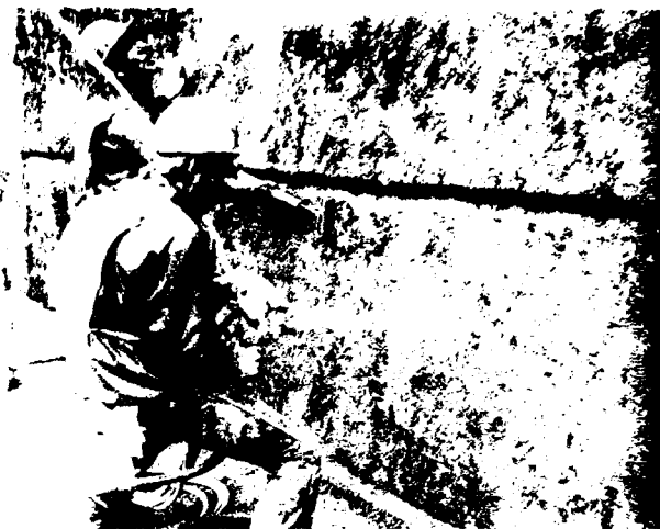
APPLICATION OF THE SPRAY-UP MORTAR AND FIBER FIBERS FROM THE "NOZZLE" AND "CUTTER HEAD" DURING THE TRIAL COATING OPERATION. ROLLING OF THE COATING IS BEING DONE IMMEDIATELY BEHIND THE SPRAY APPLICATION.
