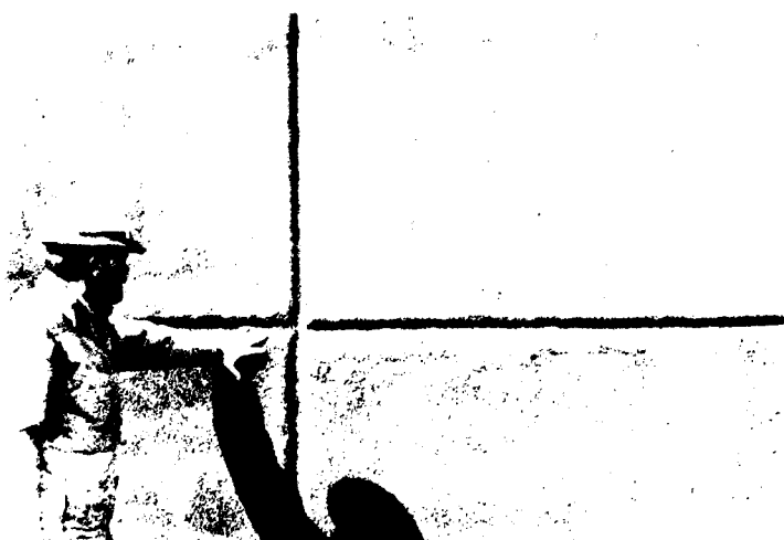
APPEARANCE OF THE WALL COATING IN THE UPPER LIFTS WHICH HAD MINIMAL DETERIORATION.
