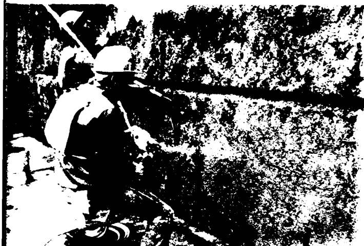
APPLICATION OF THE SPRAY-UP MORTAR AND FIBERGLASS FIBERS FROM THE "NOZZLE" AND "CUTTER HEAD" DURING THE TRIAL COATING OPERATION. ROLLING OF THE COATING IS BEING DONE IMMEDIATELY BEHIND THE SPRAY APPLICATION.
