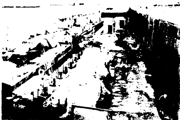
WORKING FROM BARGES TO APPLY THE LOCK WALL COATING NEAR THE UPPER LIFTS.
