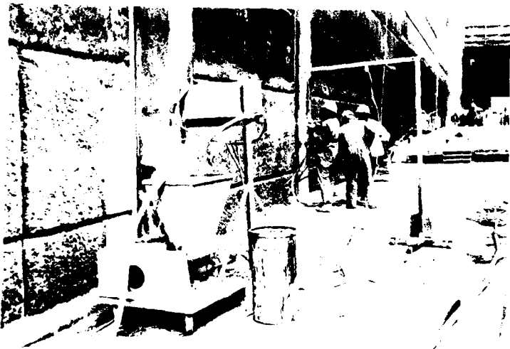
ONE OF THE FOUR SPRAY-UP UNITS. MORTAR IS BROUGHT FROM THE MIXER IN THE TUB AND DUMPED INTO THE GROUT PUMP. IT IS PUMPED THROUGH THE HOSE TO THE NOZZLE WHERE IT IS ATOMIZED AND SPRAYED ONTO THE WALL WHILE SIMULTANEOUSLY CUTTING THE FIBERS FROM A CONTINUOUS OVERHEAD STRAND AND BLOWING THEM ONTO THE WALL.
