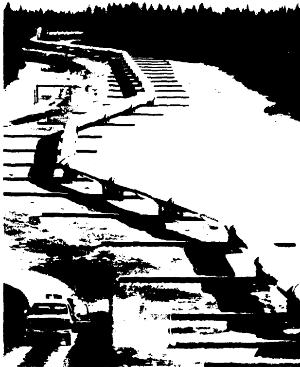
Figure 7. Special beam supports used at Denali Fault section of pipeline.
