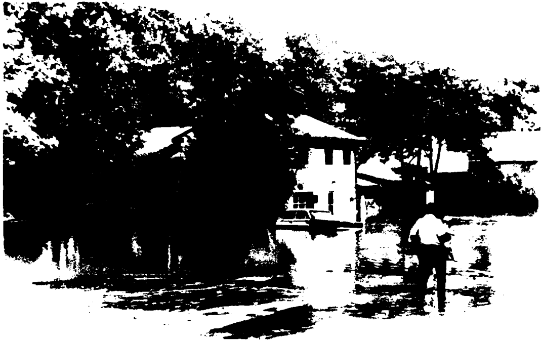
FIGURE 3 - Floodwaters from the August 28, 1971, flood surround the Valley Stream Bar and Restaurant located on Bridgetown Pike. (Photo from September 2, 1971, issue of Delaware Valley Advance ).
