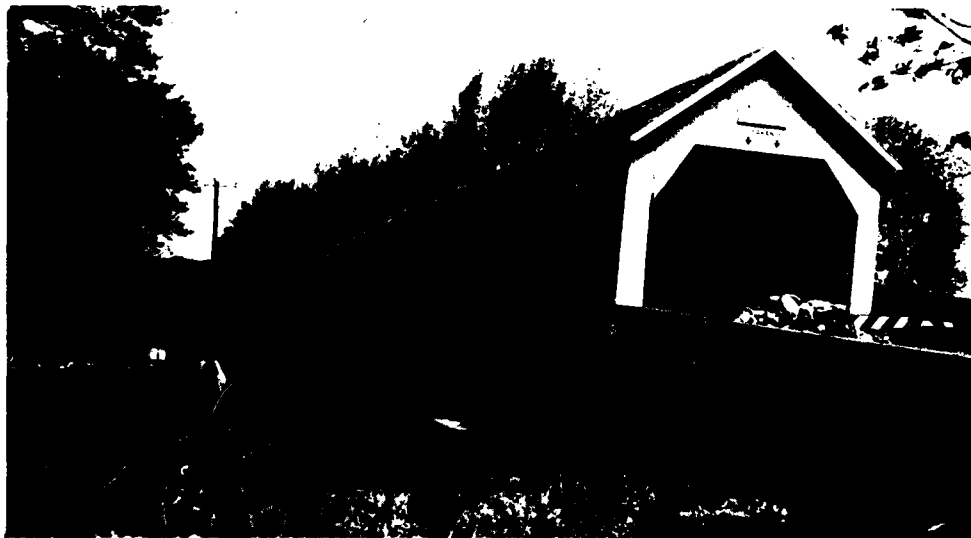
Figure 3.--BRIDGES ACROSS EAST BRANCH PERKIOMEN CREEK Top view is the upstream side of Main Street bridge in Sellersville. Bottom view is Moods covered bridge at Mile 6.89.
