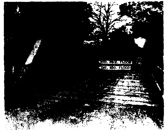
Photograph shows possible future flood heights at Bucks Road bridge.
