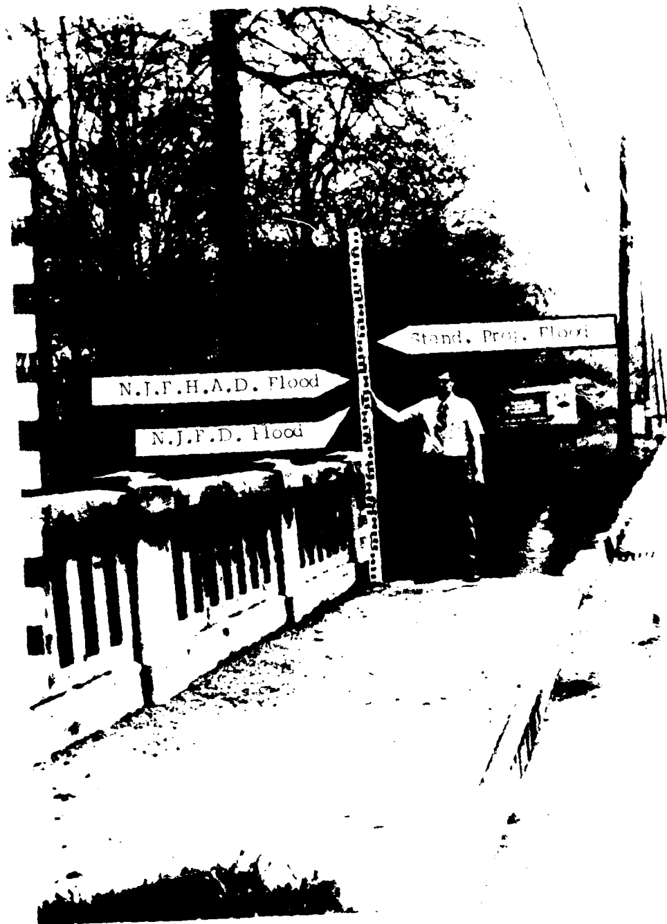
FIGURE 11 - Future flood heights at Delsea Drive (N.J. Rt. 471) bridge on Mantua Creek
