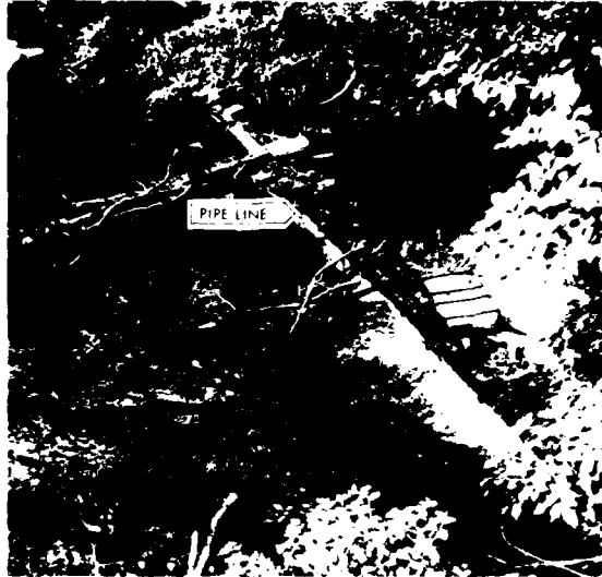
FIGURE 1 - Accumulated debris at a pipe line crossing Crum Creek upstream of MacDade Boulevard.
