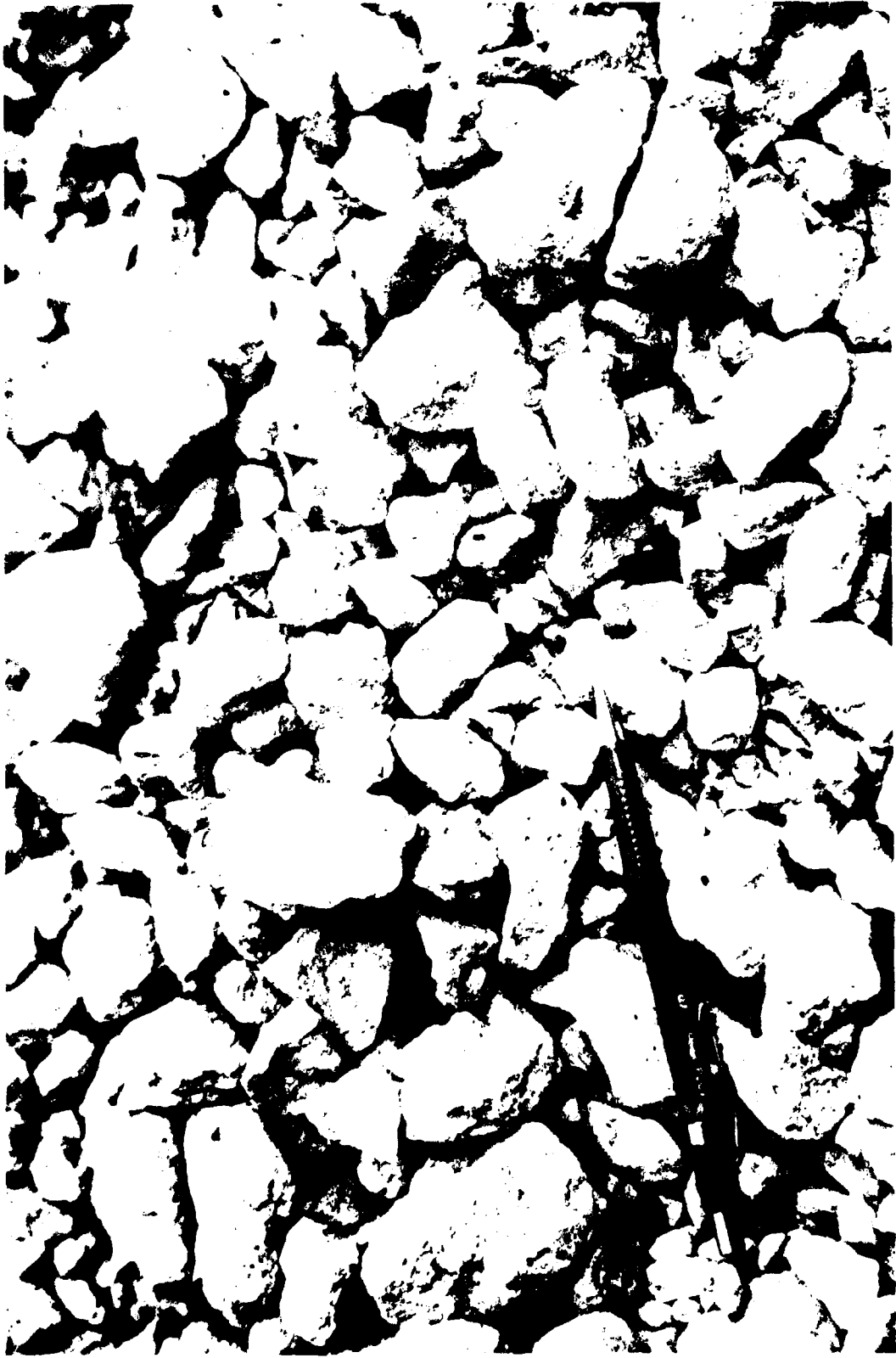
Figure 8. Stockpiled excess material obtained from crushing the old PCC pavement at Jacksonville International Airport.
