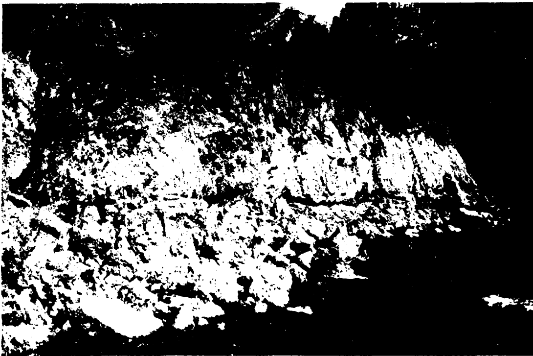
Figure 3 Johnson Creek Bank Failure Due to Undermining.
