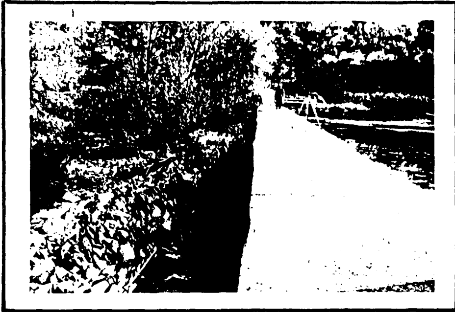
DOWNSTREAM ROCK PROTECTION OF SPILLWAY - NO. 4
