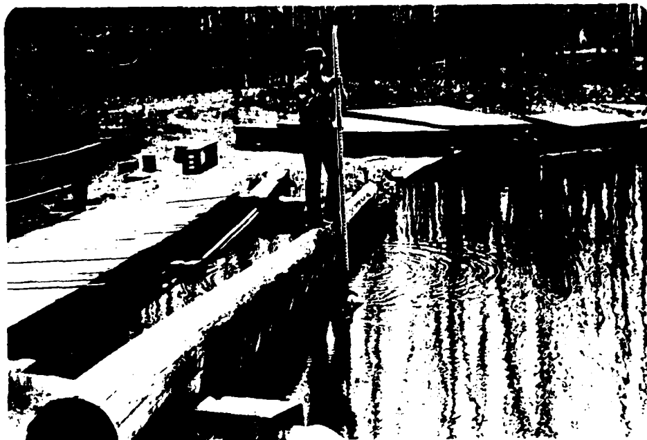
C. Spillway Approach
