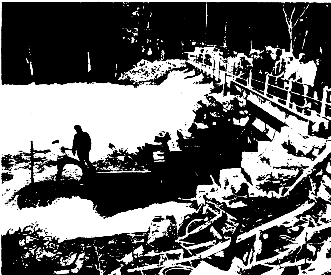
Figure 1 Workmen prepare to place large boulders in an attempt to reinforce a pier of the state dam at Owasco Lake outlet. Photo taken 25 June 1972.
