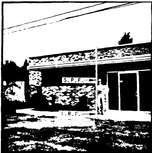
Figure 41- Arrows indicate the depth of flooding for the Standard Project and Intermediate Regional Floods at the Ellicott Creek Volunteer Fire Company house upstream of Niagara Falls Boulevard, creek mile 3.45 in the town of Amherst.
