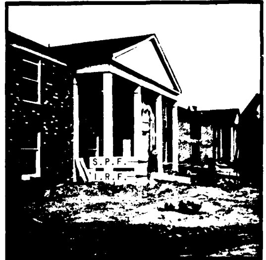
Figure 44- The heights of the Standard Project and Intermediate Regional Floods are indicated by arrows at the Sturbridge Village Apts. under construction at approximate creek mile 9.3 in the town of Amherst.
