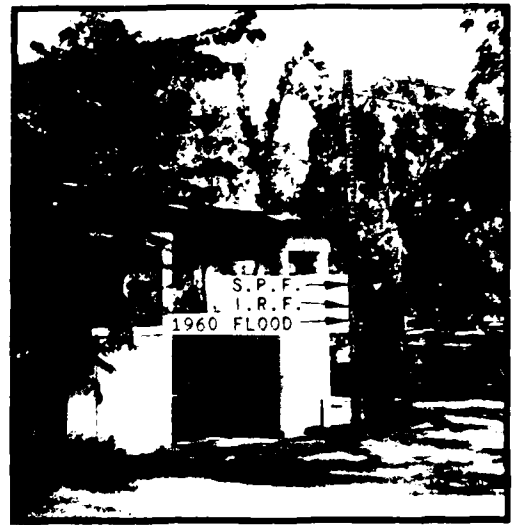
Figure 46- The Standard Project, Intermediate Regional and the 1960 flood heights are indicated by arrows at Walker's Grove just downstream of Wehrle Drive near creek mile 14.0 in the town of Amherst. Although depth of flooding is great, damages would be minor.
