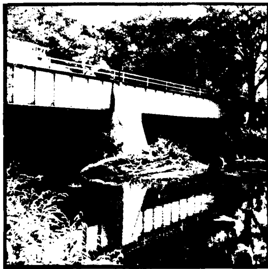
Figure 13- Photo of upstream side of Maple Road bridge. Note amount of debris collecting at center pier.
