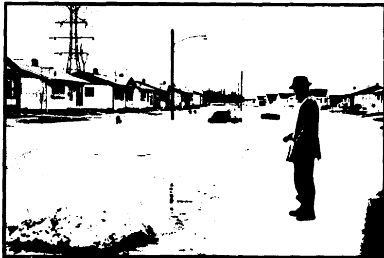
Figure J- Photo showing flooding conditions on Frederick Road in the city of Tonawanda, near creek mile 1.5, during the January 1959 flood.
