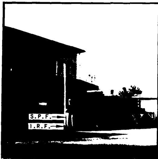
Figure 48- The heights of the Standard Project and Intermediate regional Flood heights are indicated by the arrows at the residence located just downstream of Harris Hill Road, creek mile 18.35 in the town of Lancaster.
