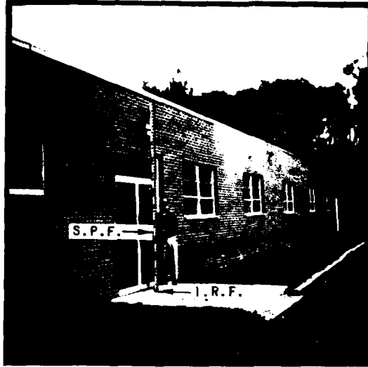
Figure 47- The Standard Project and Intermediate Regional Flood heights are indicated by the arrows at the Bowmansville Volunteer Fire Company House, near creek mile 17.8 in the town of Lancaster.
