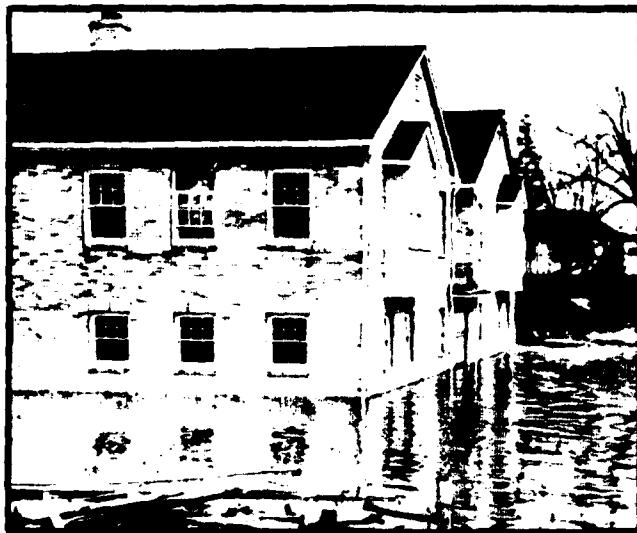
Figure H- Photo showing flooding conditions on the grounds of St. Rita's Convalescent Home for Children, Millersport Highway near North Forest Road, town of Amherst, at creek mile 7.4 during the April 1940 flood.
