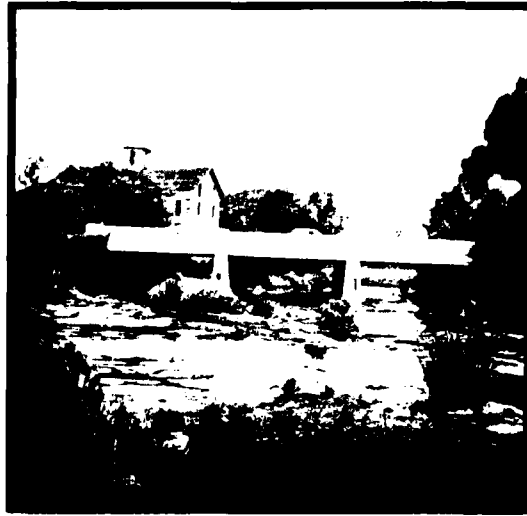
Figure 11- Photo looking at upstream side of Millersport Highway bridge.
