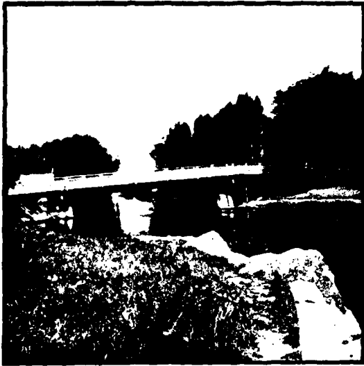
Figure 22- Looking downstream toward the Fremont Street bridge at creek mile 0.44 in the city of Tonawanda.
