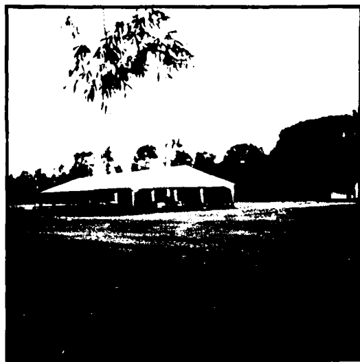
Figure 21- Looking at shelter within flood plain at Bowmansville Volunteer Fire Company Grove. Photo indicates wise flood plain usage.
