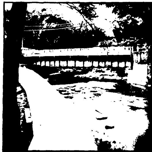
Figure 25- Looking downstream at the Glen Avenue bridge at creek mile 12.9 in the village of Williamsville. This bridge constructed in 1937 after the 1936 flood washed out the existing structure.
