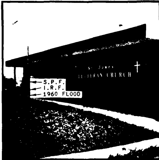
Figure 43- The relative flood heights of the Standard Project, Intermediate Regional and 1960 flood are indicated by arrows at the St. James Lutheran Church, approximate creek mile 9.15 in the town of Amherst.
