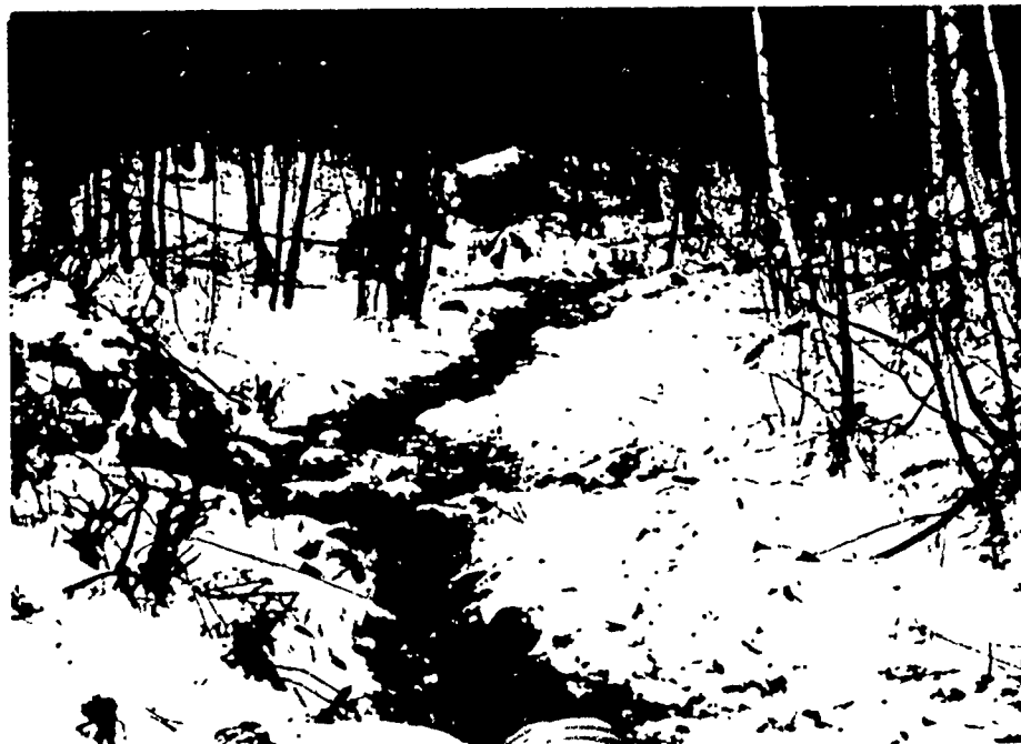
12. Spillway discharge channel downstream of road (10 Mar 81).
