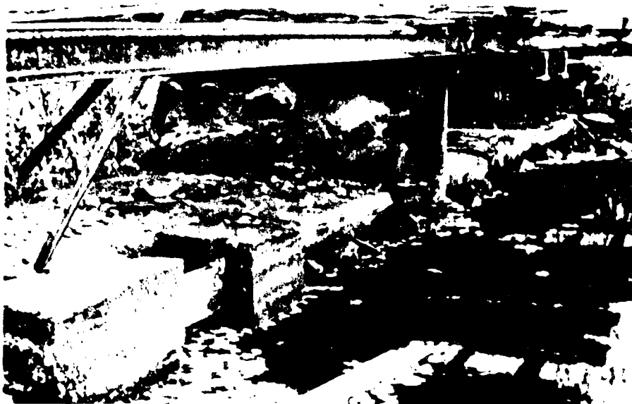
6. Spillway crest, bridge and drop inlet. Note undermining of crest slab. Iron pipe at center of crest is control for sluiceway gate.
