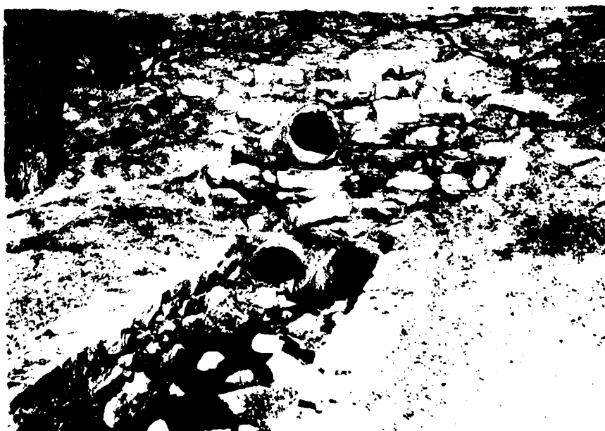
PHOTO 4 DOWNSTREAM END OF SPILLWAY DISCHARGE CULVERTS
