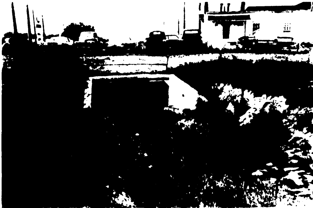
FIGURE 4 - Vegetation obstructs the channel upstream of a box culvert across Trout Creek. Culvert is located in the vicinity of 4th and Brookdale Streets.
