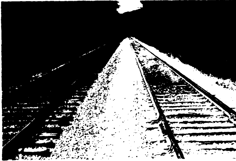
Crest of railroad embankment looking north from Powder Mill Road crossing.
