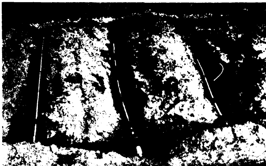
Figure 27. Slotted collector pipe in trenches (test section 2)
