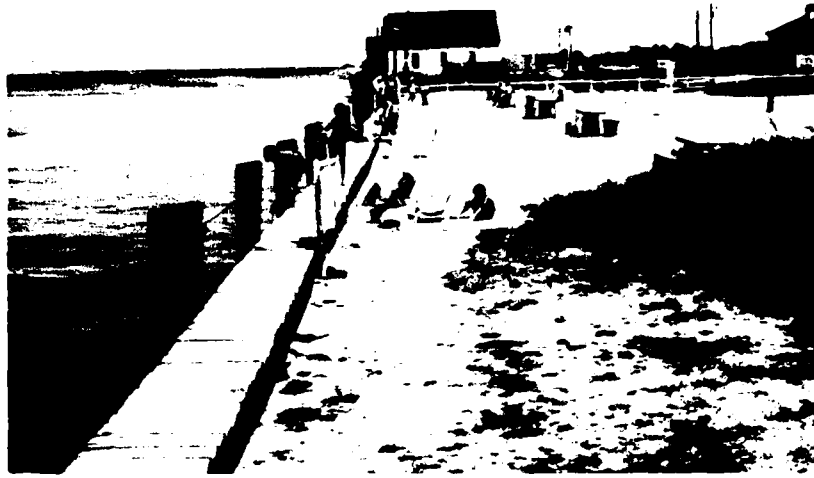
THE BULKHEAD AT THE EAST BOAT BASIN
