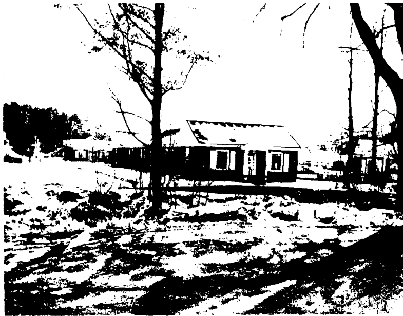
Melrose Terrace Housing Development for Elderly, looking downstream. Standard Project Flood will overtop bank in foreground to a depth of as much as five feet.
