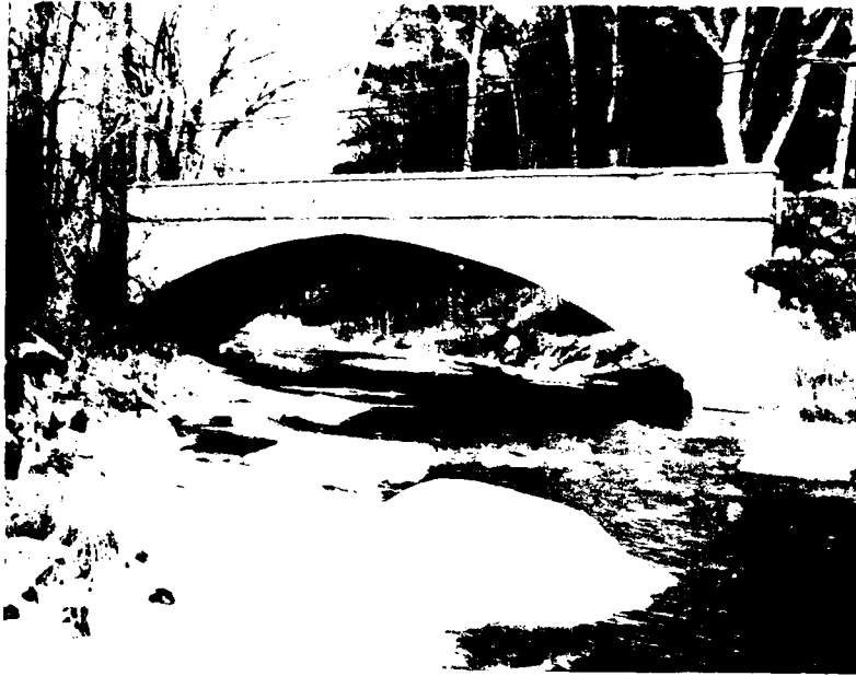
State Highway 9 bridge over Whetstone Brook. Standard Project Flood will overtop bridge deck by about three feet.
