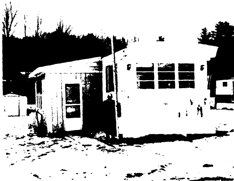
Flood Heights, mobile home, in Mountain home Trailer Park, right bank Whetstone Brook just downstream from Mountain Road, West Brattleboro.
