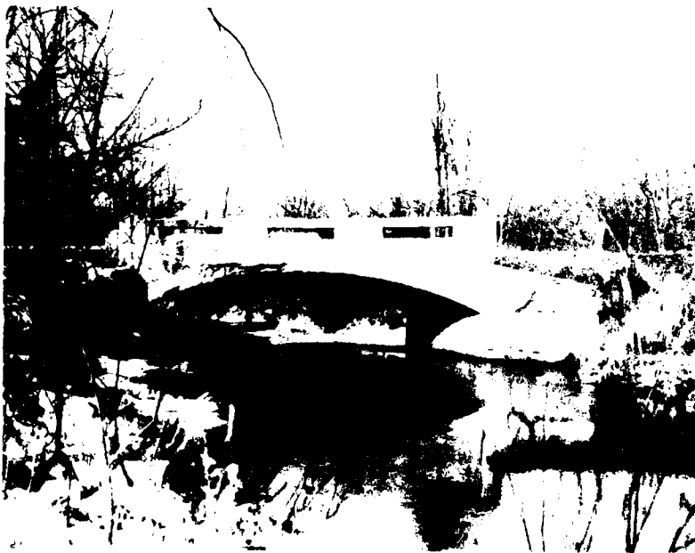
Meadowbrook Road bridge. Both Standard Project and Intermediate Regional Floods will overtop this bridge deck.
