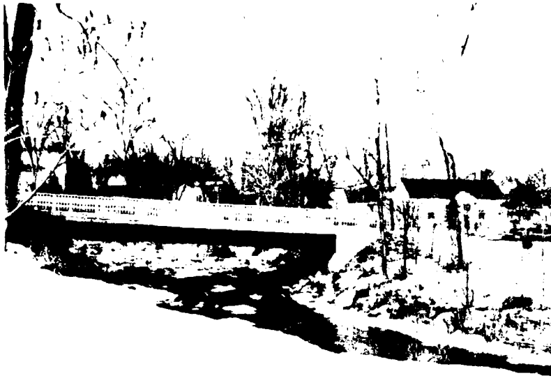
George F. Miller Drive bridge over Whetstone Brook. Entrance to Melrose Terrace housing development. Considerable flow will bypass this bridge through area in vicinity of cars.
