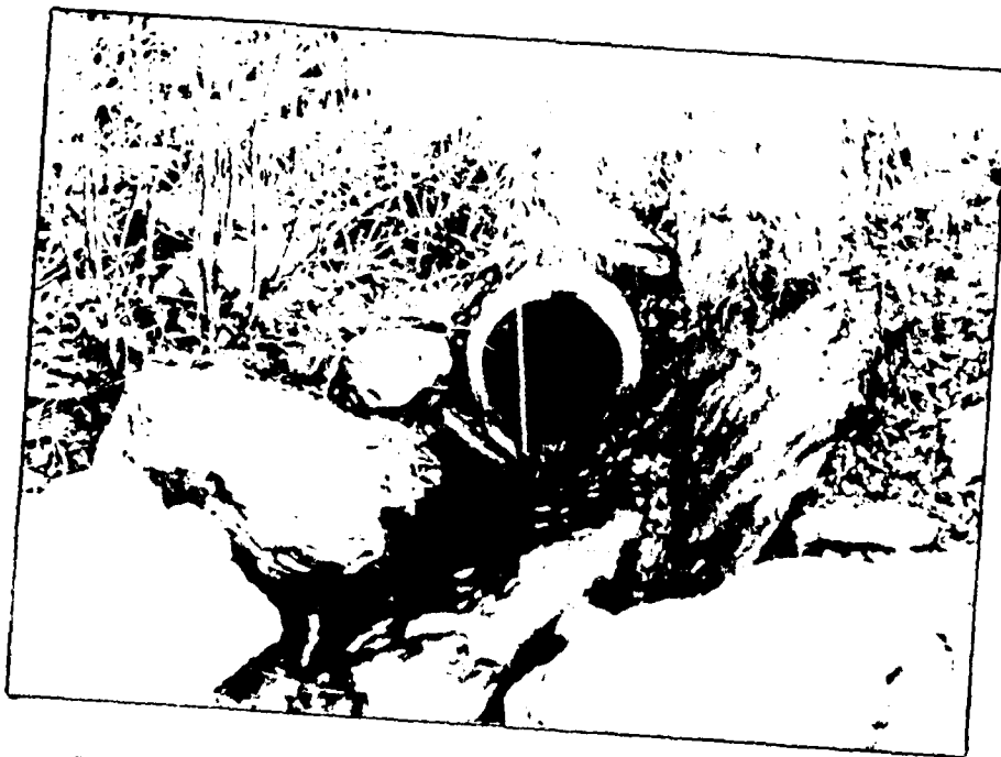
PHOTO 8. Close-up View of Downstream End of Outlet Conduit
