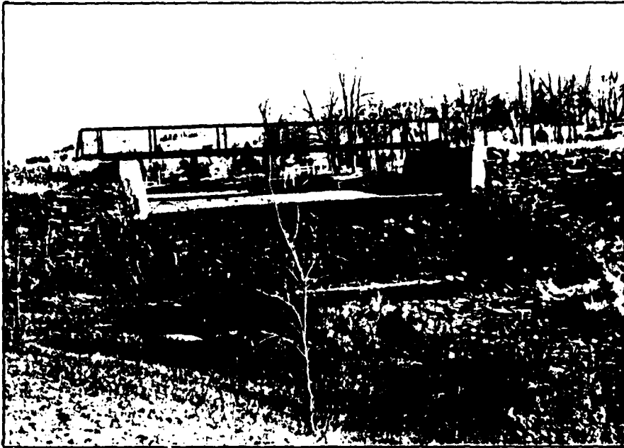
PHOTO 3. View of Downstream Side of Spillway
