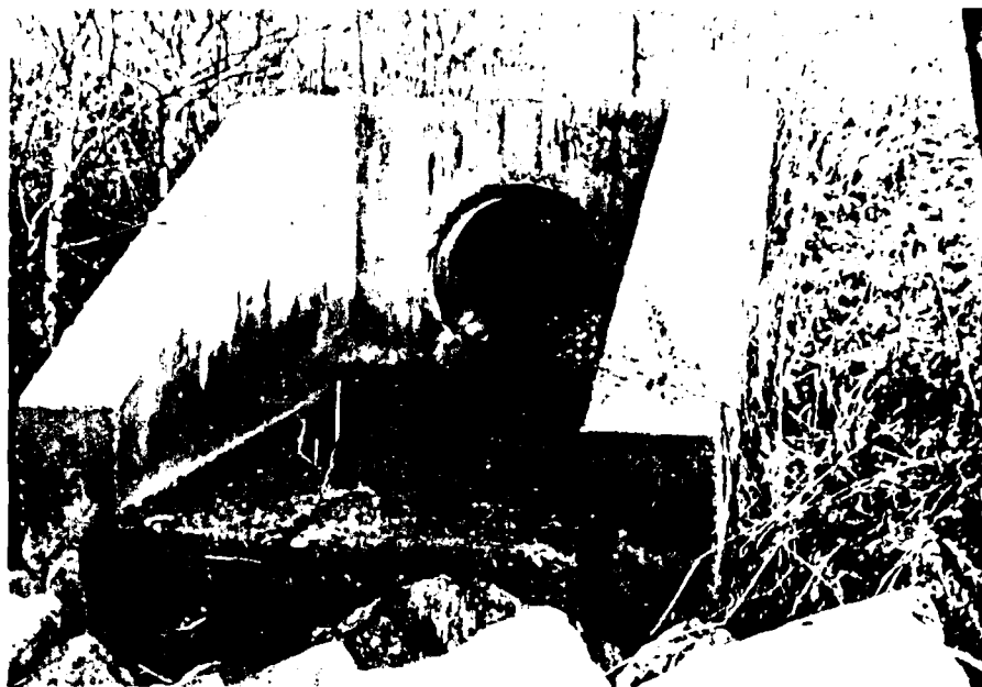
9. Downstream end of outlet conduit and headwall.
