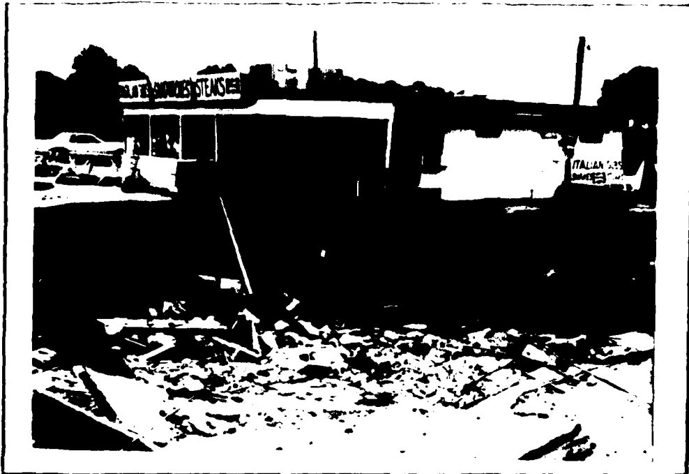
5. VIEW EXHIBITING UNDERMINING OF RESTAURANT DOWN- STREAM OF THE RIGHT ABUTMENT. AUTO IN LEFT BACKGROUND IS TRAVELING UPON U.S. ROUTE 13. (8/12/80)
