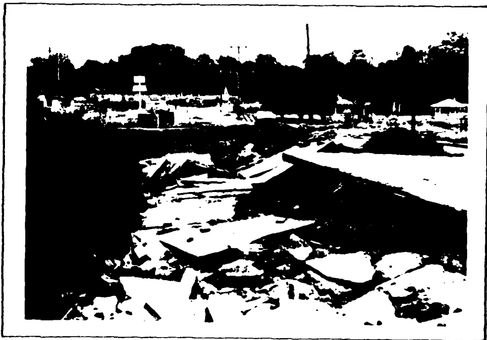
6. VIEW OF FAILURE ZONE LOOKING TOWARDS RIGHT ABUT- MENT. AREA OF OVERTOPPING EXTENDED ABOUT 500 FEET TO CEMETARY IN BACKGROUND. (8/12/80)
