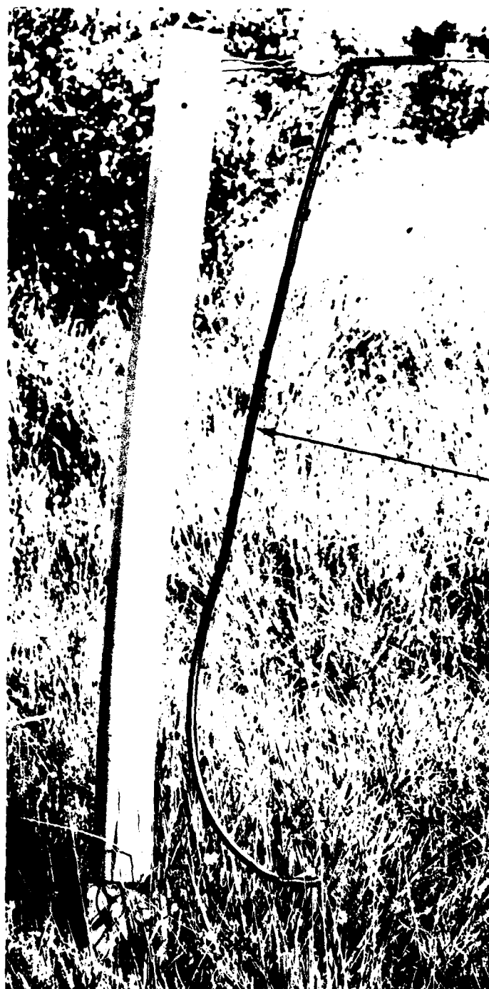
Fig 17 Photograph of beverage showing terminating resistor
