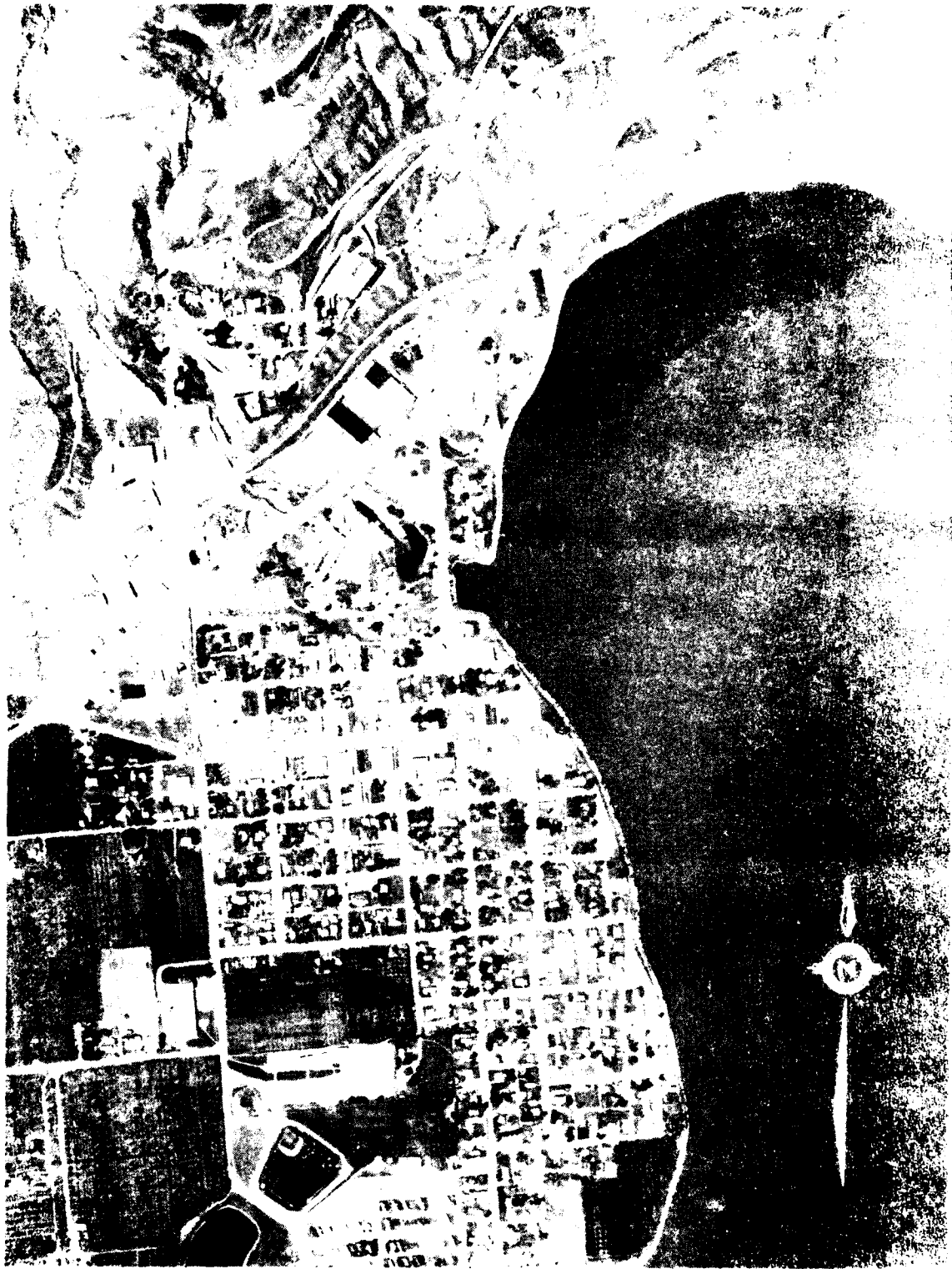
FIGURE 12. AERIAL PHOTOGRAPH OF BREWSTER, WASHINGTON, 1974. IMPACT: MAY 1974. SCALE: 1" = 800' ±
