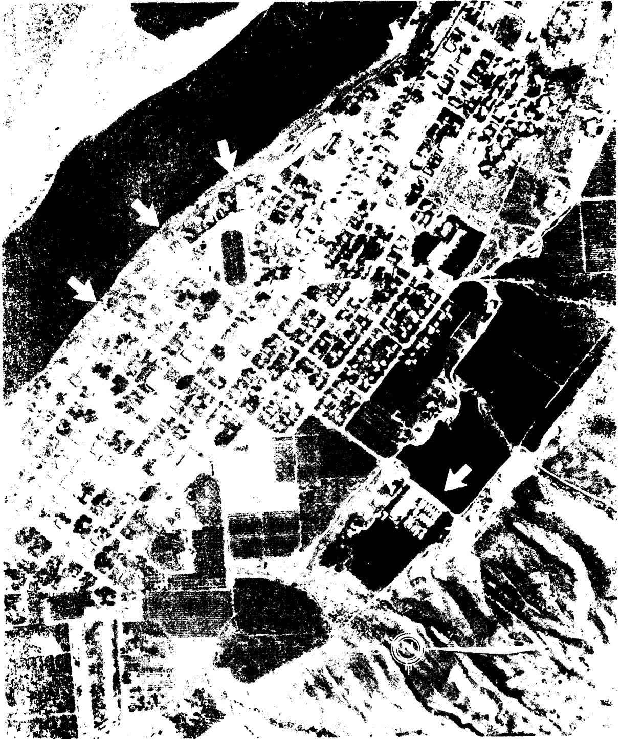
PHOTOGRAPH OF SEATTLE, WASHINGTON, DURING PHASE I OF THE CITY'S DEVELOPMENT. SEPT. 1977.
