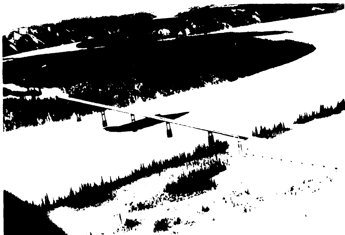
Figure 3. Aerial view of Yukon River Bridge.
