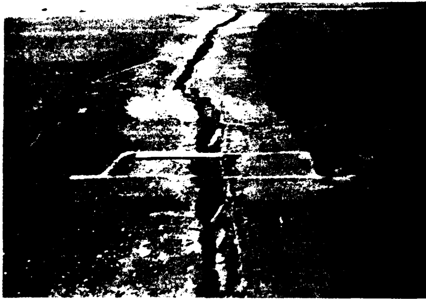
(a) Pavement before cut showing 4-inch wide crack.
