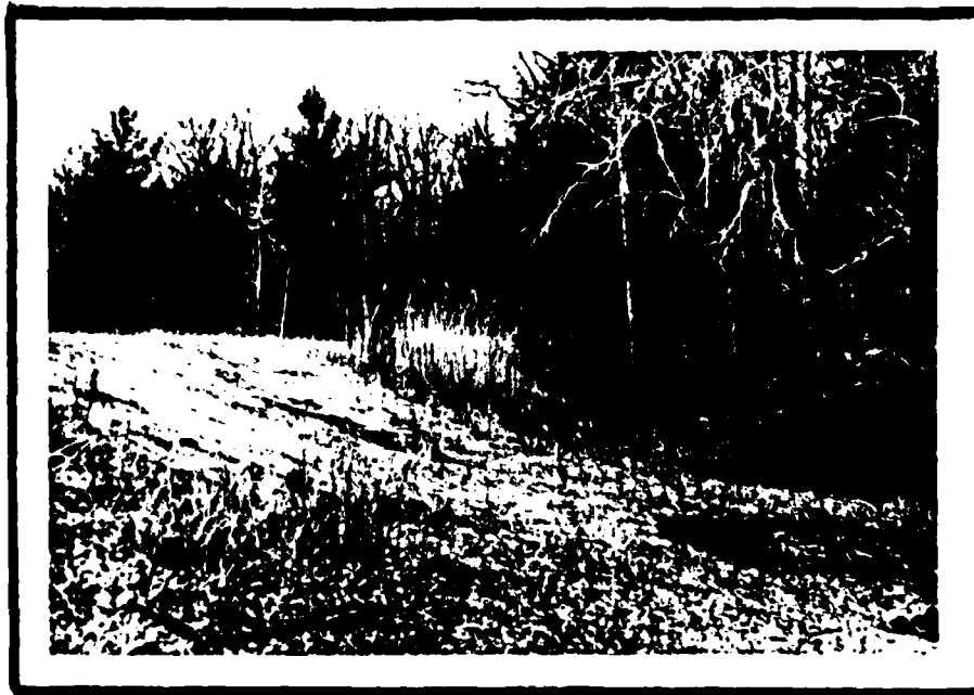
LEFT END DOWNSTREAM SLOPE - NO. 3
