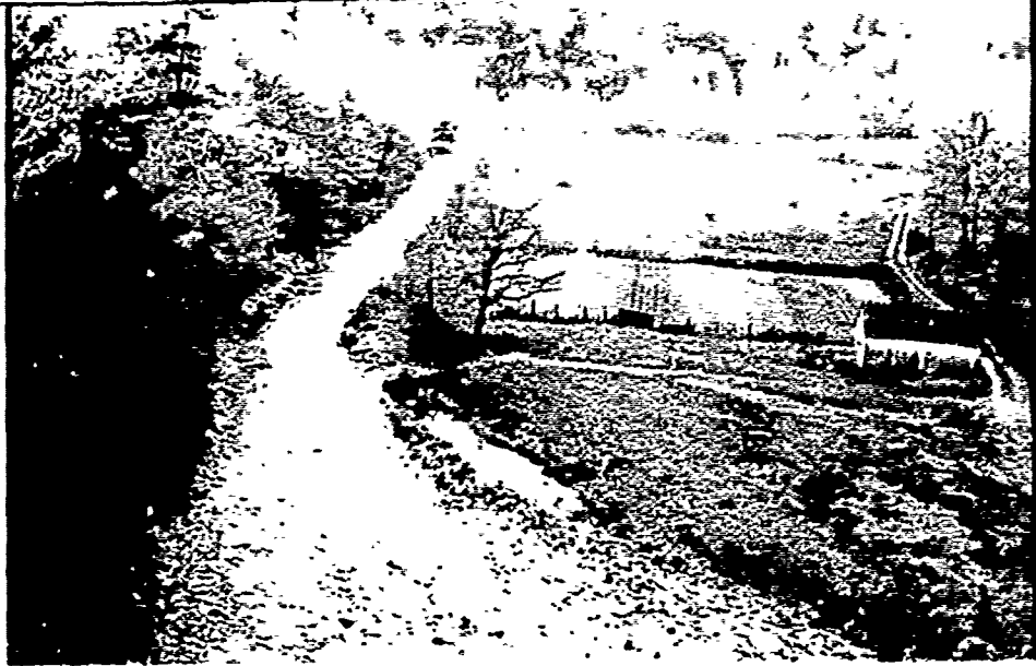
PHOTO # 5 DOWNSTREAM AREA
